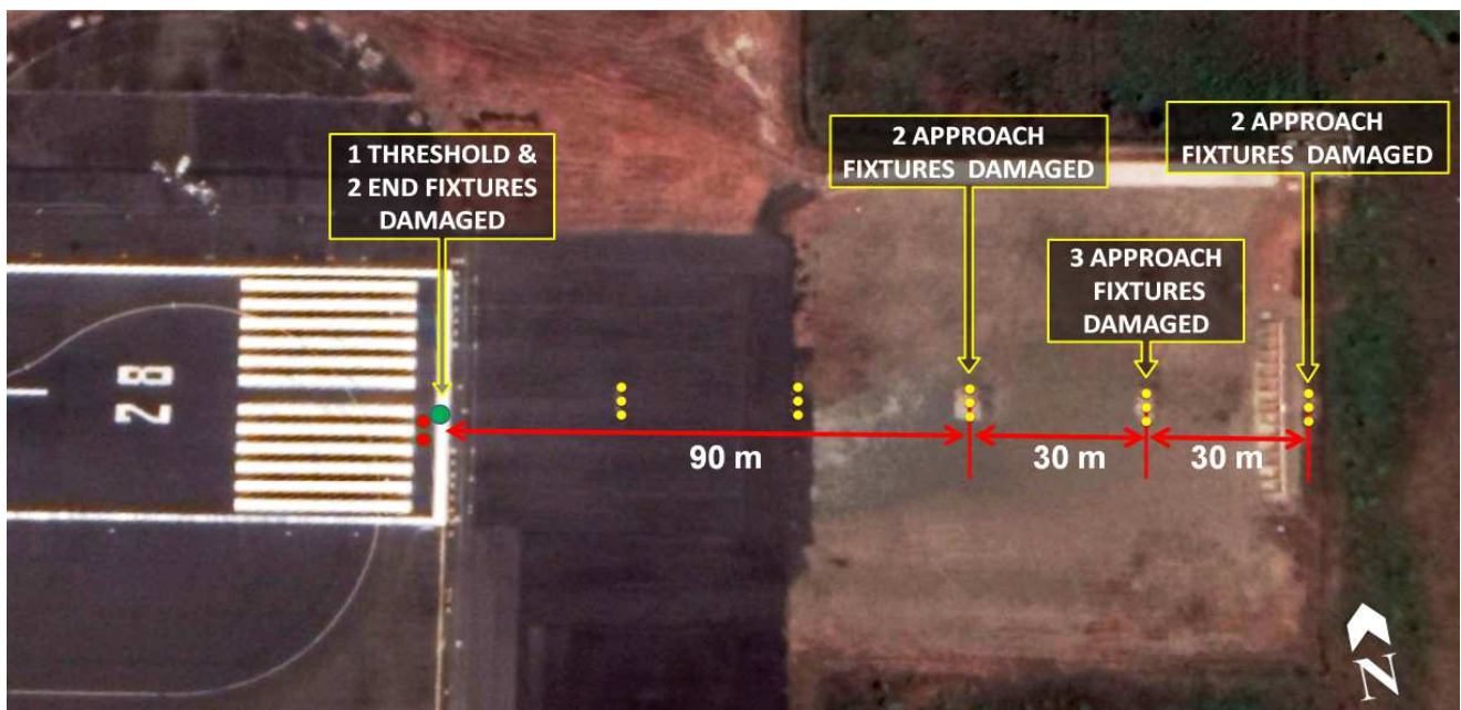
Figure 3: The location of the damaged lights in RESA.
